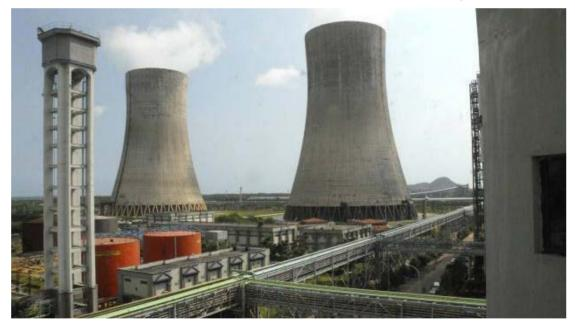
Figure 2. Hyperboloid Cooling Towers installed in a thermal Power Plant
