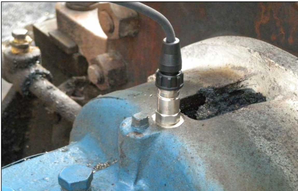
Figure 2 – General Purpose Accelerometer Mounted on a Centrifugal Pump sending vibration signal to a nearby EchoPlus® Wireless Junction Box
