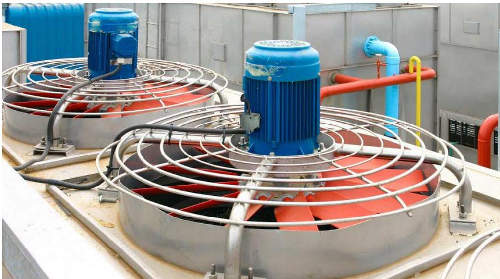
**Figure 8 Electronic Vibration Switch mounted on a Cooling Tower Motor**
