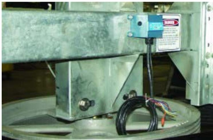
**Figure 5 Mechanical Vibration Switch installed on a Cooling Tower Fan**
