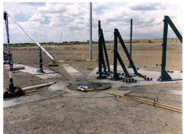
A typical blast sensor installation requires long cables for signal transmission. Data acquisition equipment may be thousands of feet away.
