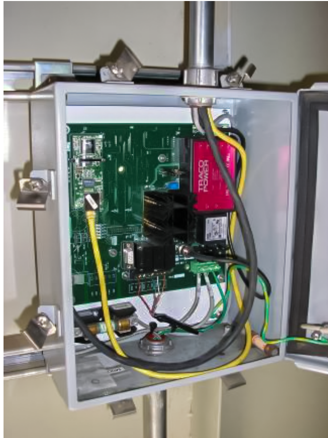
Figure 7 EFREM Receiver Mounted on Exciter Cubicle Wall
